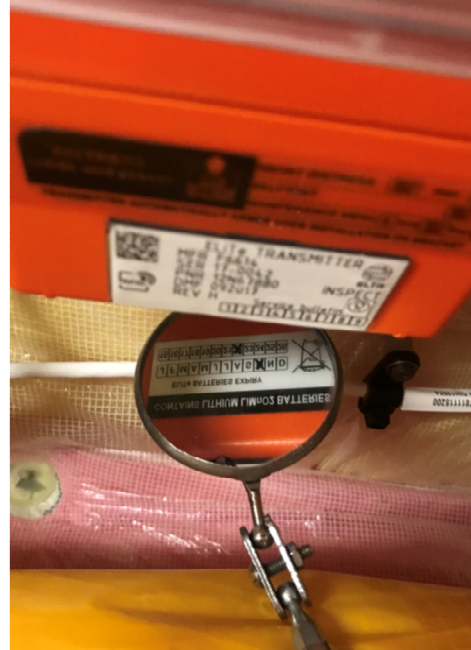
Figure 8: Fixed ELT Battery Marking
